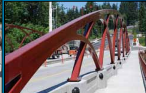
May Creek Bridge Redmond, WA.
