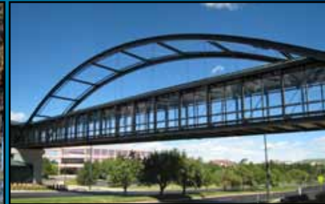
Dry Creek Bridge Denver, CO.
