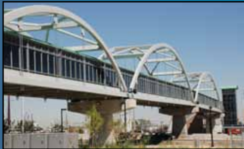
Hwy 36 Bridge Denver, CO.
